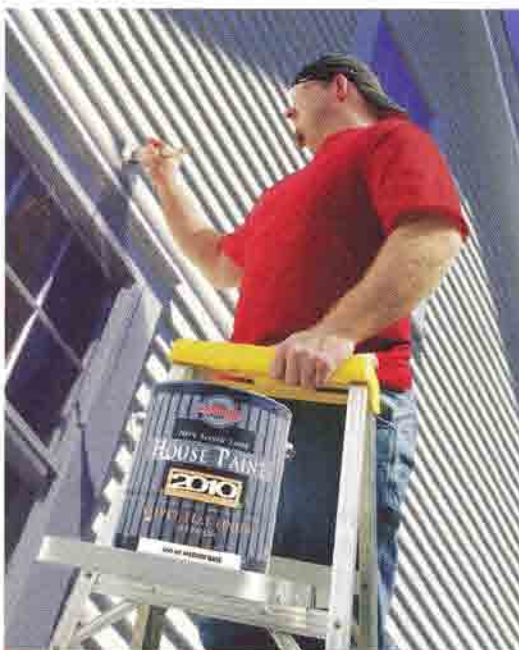
HIGH SCORER The flat-finish California 2010 paint, while on the pricey side at $38 a gallon, looked best overall after years of exposure.
