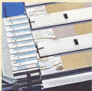
RACKED WITH PAINT Our rooftop tests mimic nine years of weathering.
